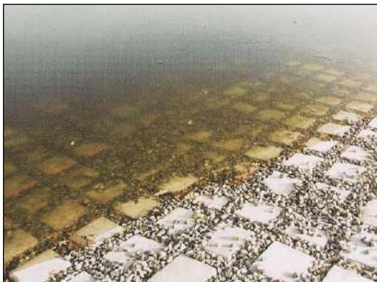
Figure 7:5 - Subsea Cable Covered in Concrete (Cable Concrete, 2004).
