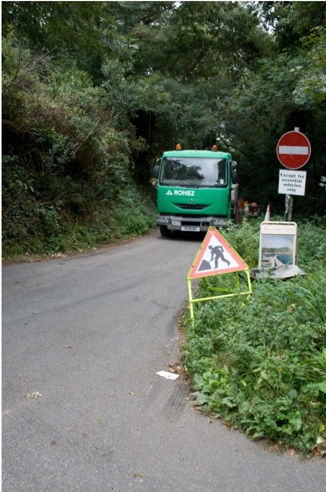
Figure 6.2.4 Saints Bay access road
