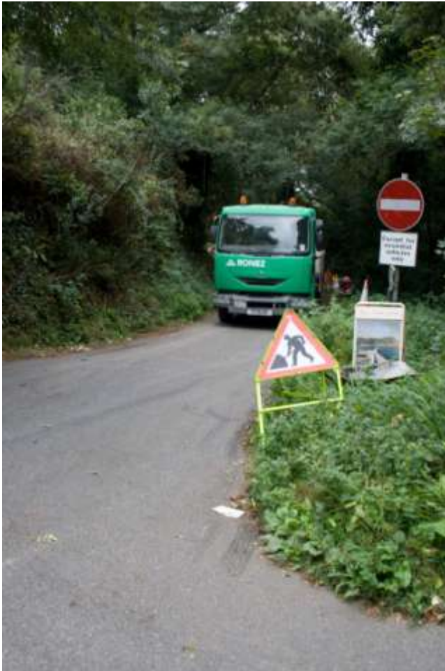
Figure 6.2.4 Saints Bay access road
