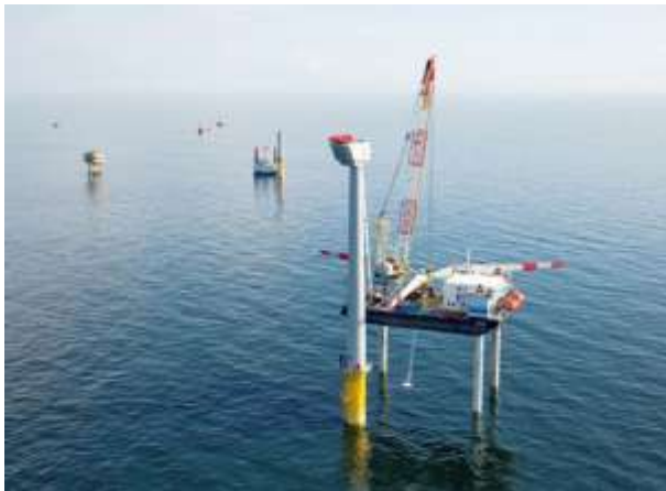
Figure 26 :Jack-Up Barge installs Germany's first offshore wind turbine (source MarineLog)
