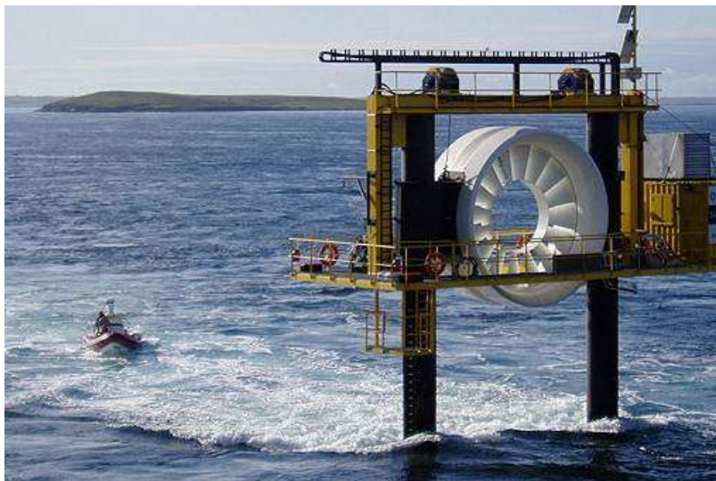
Figure 59 : OpenHydro Prototype Device (source OpenHydro)
