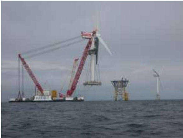
Figure 28 : Installation of jacket and 5mw wind turbine generator at the Beatrice Offshore Windfarm (source SCALDIS SMC)
