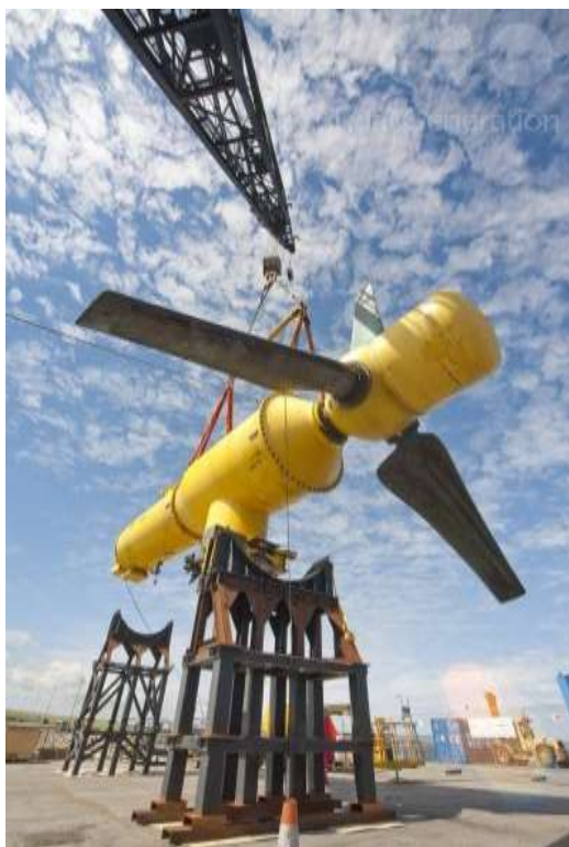
Figure 60 : Deployment of Tidal Generation Device (source - Tidal Generation Limited)
