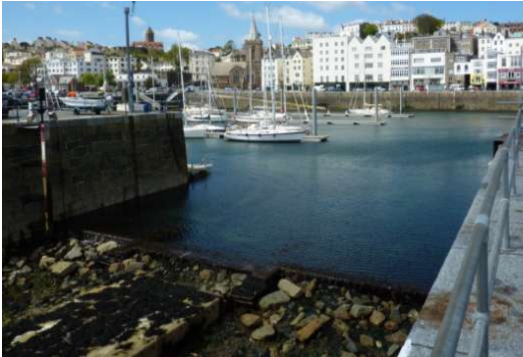
Figure 2: Victoria Marina - silt and debris at sill
