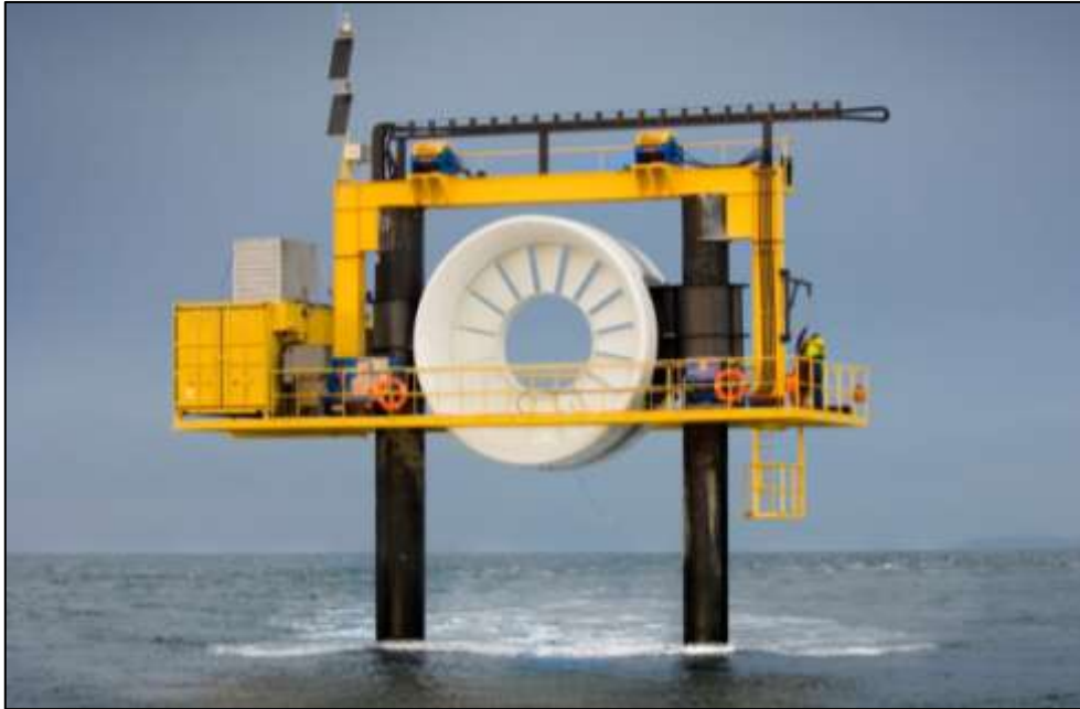
Figure 7: OpenHydro test rig 11
