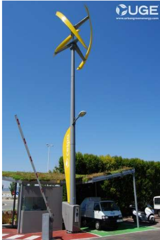
Figure 46: Urban Green Energy Vertical Axis Turbine used as part of car parking infrastructure, advertising space and for lighting
