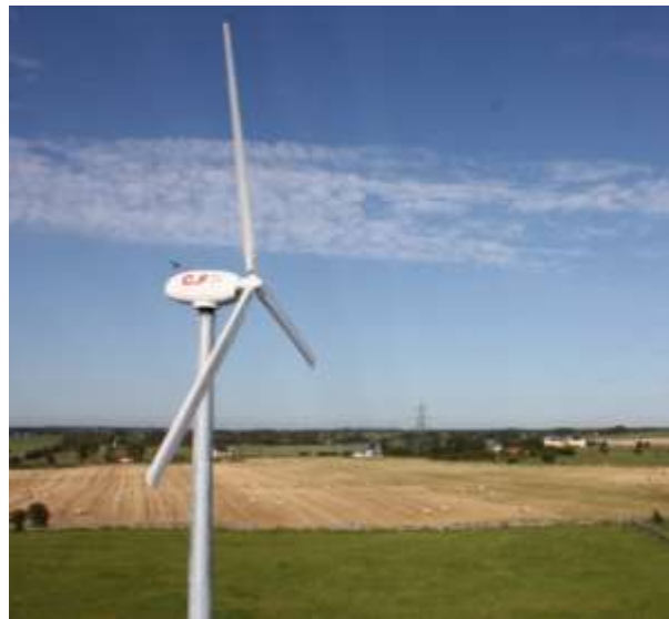
Figure 49: The C&F 50e 50 kW wind turbine 86
