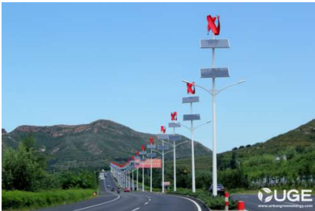
Figure 47: Urban Green Energy PV and wind integration system for street lighting
