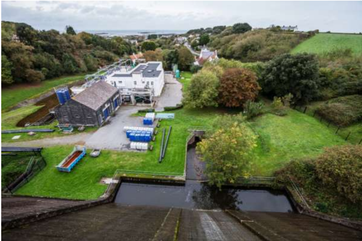
Figure 12: St Saviours treatment works 22
