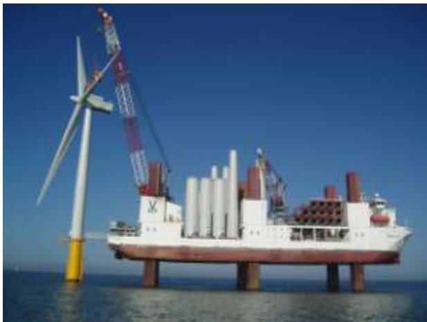
Figure 2.9 – MPI Resolution installation vessel completing installation of an offshore turbine (photo - Courtesy of MPI)
