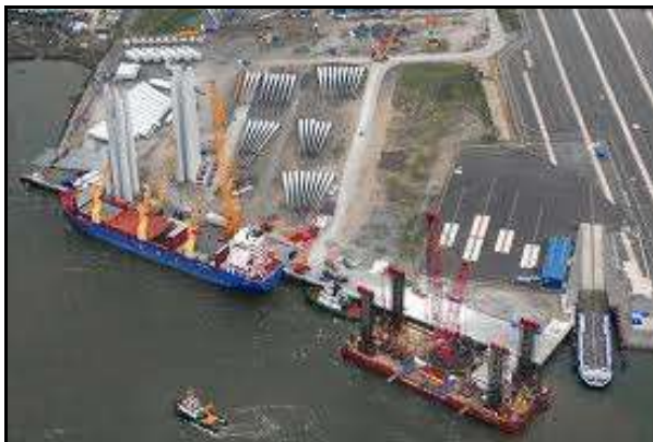
Figure 2.10 – Port of Mostyn turbine pre-assembly area (photo – courtesy of Port of Mostyn)
