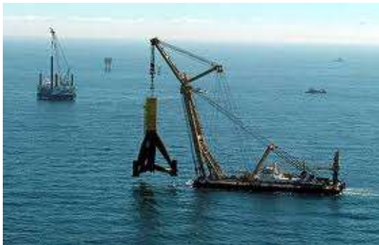
Figure 2.6 – Multibrid tripod foundations being installed (photo – Recharge 22 )
