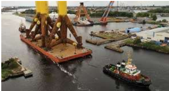
Figure 2.6 – Multibrid tripod foundations being installed (photo – Recharge 22 )
